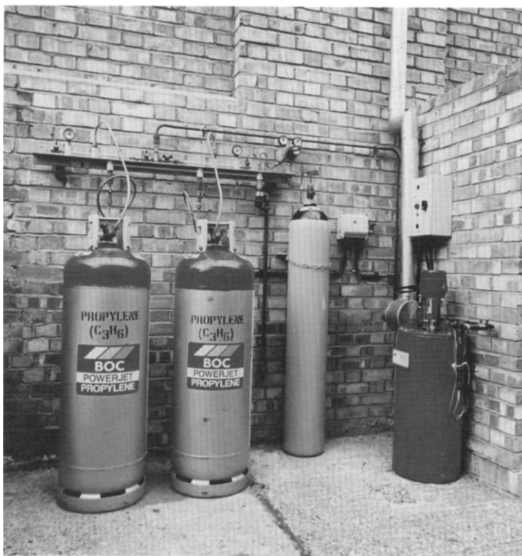
4.22 Liquid withdrawal propylene installation for HVOF (courtesy of BOC Gases).
